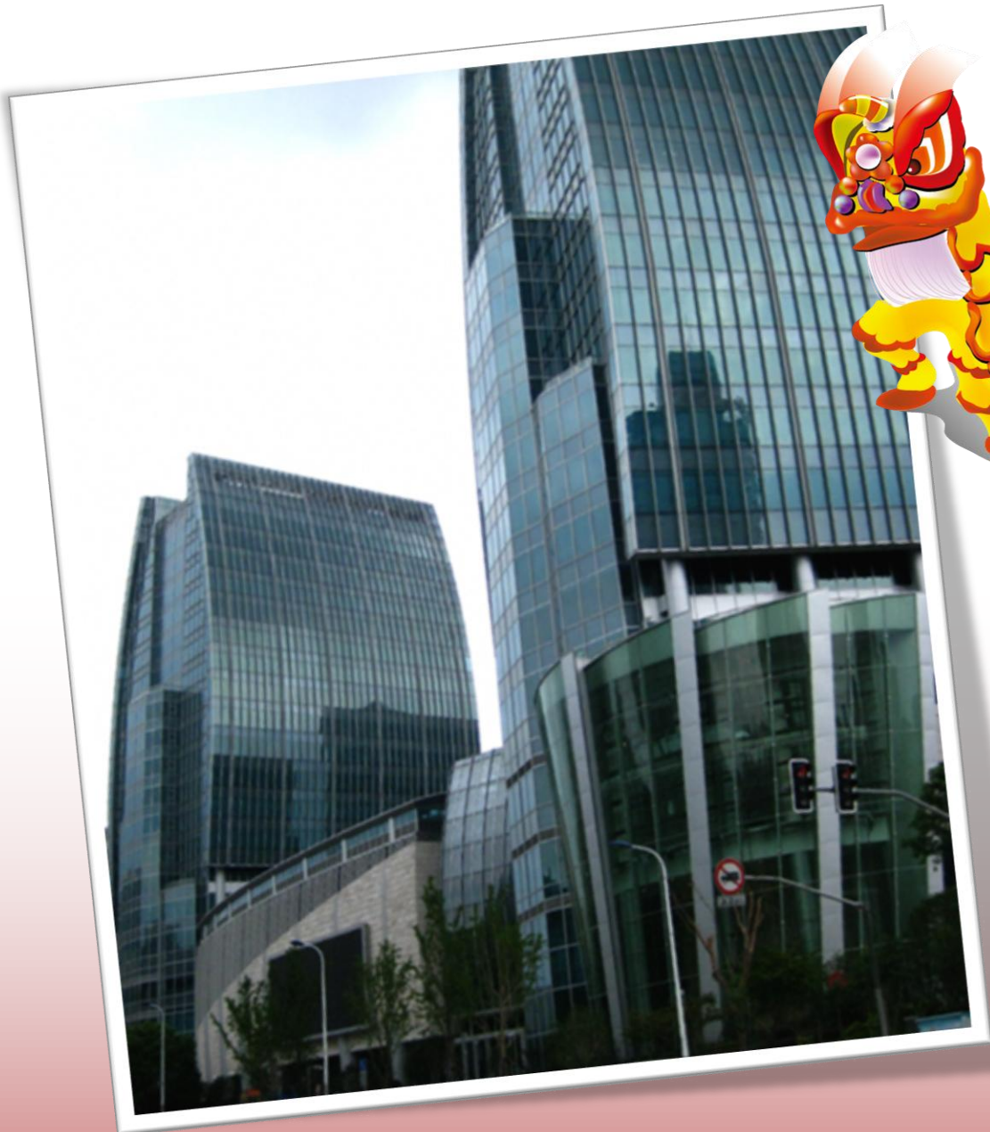
Technical Site Visit to Data Centre of Industrial Security Company, Dingxiang Road
